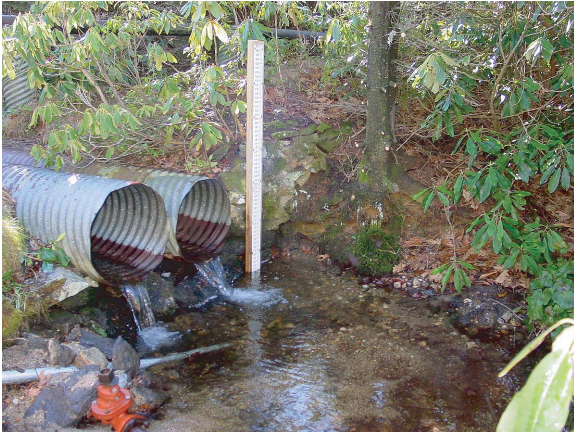
Figure 4. The downstream side of the double corrugated metal pipe (CMP) culvert where the U.S. Geological Survey gaging station was located at the Mt. Pisgah campground.
