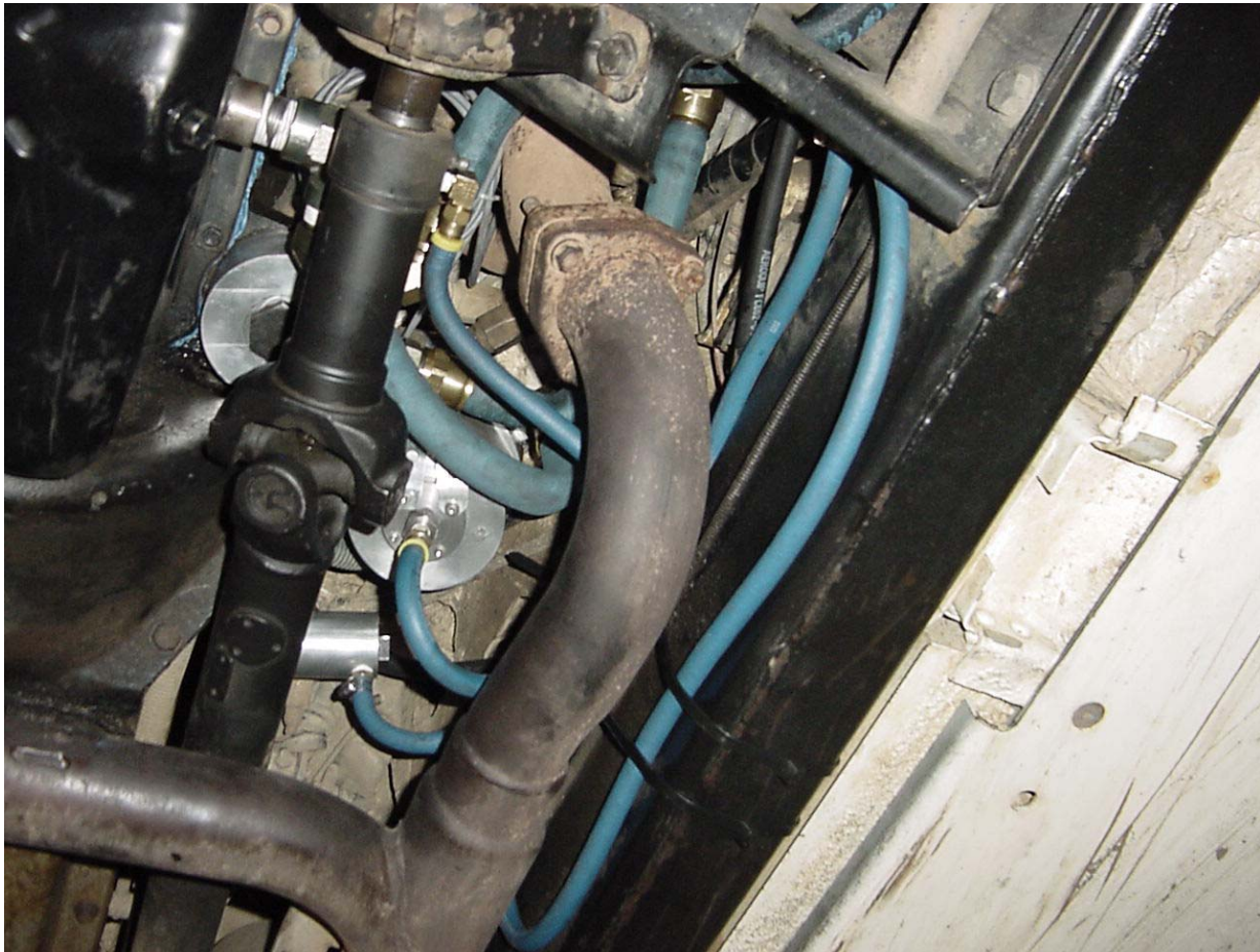
Figure 27: Filter installed in the Hummer Vehicle
