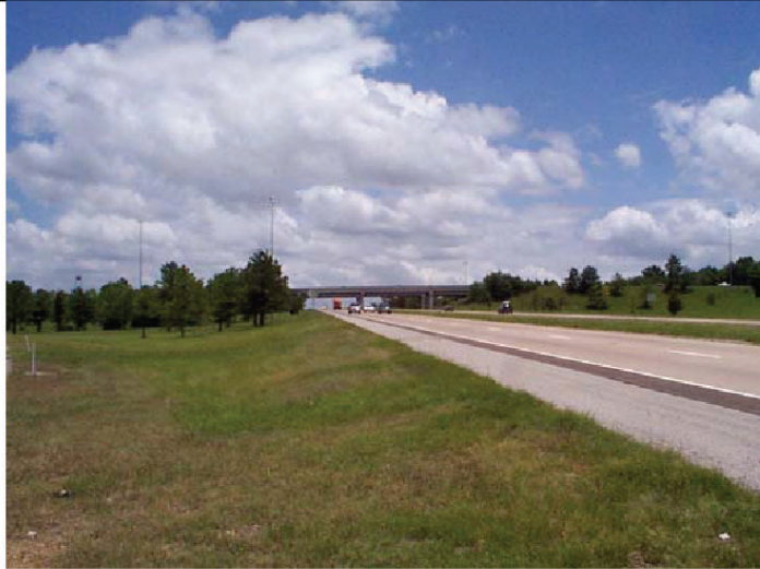
Get as close to the bridge as possible. This is too far away.
