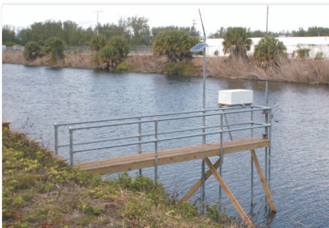
Figure 3. Turbidity probe installation upstream of structure S-155.
