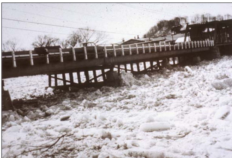
Figure 2. Bridge Street Bridge, White River Junction, Vermont, 1969.
