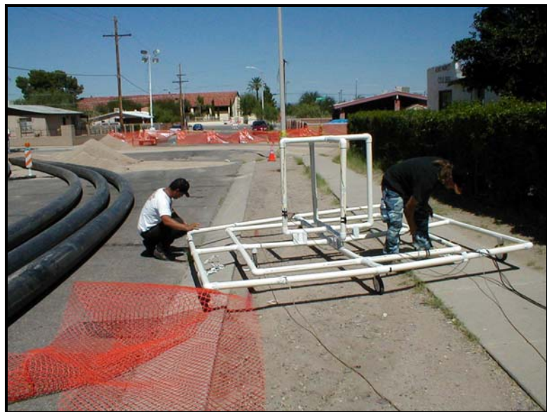
Figure 2.3: A large (3m x 3m) DNT antenna array mounted on caster wheels. The antenna system includes a 3-axis receiver antenna array. It is being used to detect failures in a large concrete sewer main in Tucson, Arizona (October, 2002)
