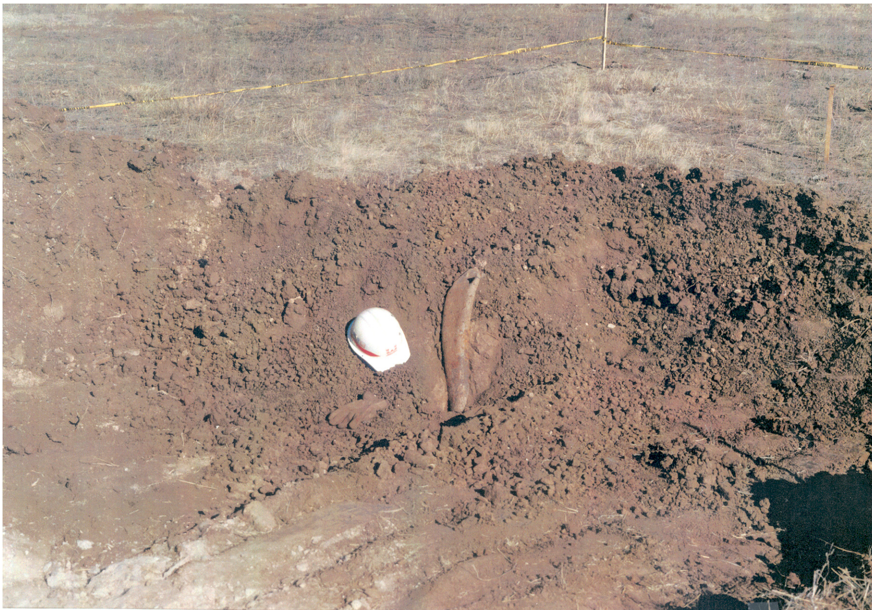
Figure 13. Excavated well casing at homestead site HL-5, former Pantex Ordnance Plant and Texas Tech Research Farm near Amarillo, Texas. Photograph by John S. Ebling.
