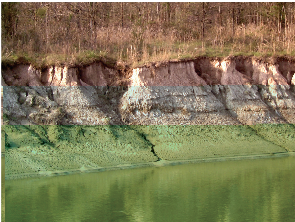
Figure 1. Downcutting by the stream channel can reduce flooding and lower the water table on the former adjacent floodplain
