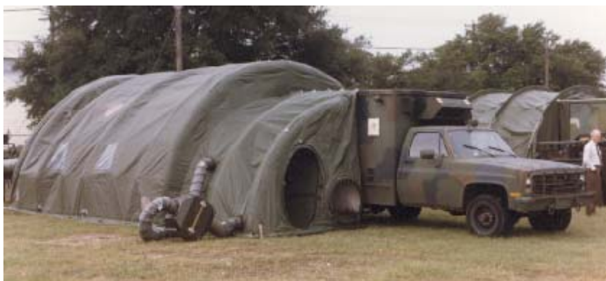
Figure 4. Air-Supported Battalion Aid Station.
