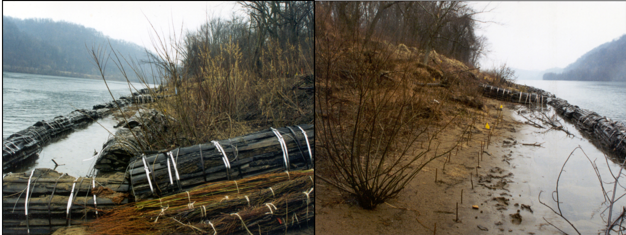
Figure 12. Slab bundles at Bat Grape Island. Notice second bundle placed landward of riverward bundle in left photograph and plantings in right photograph
