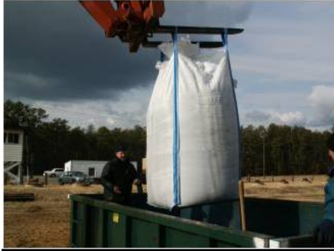
Figure 20. Emptying Super-Sacs of Granular Rubber.
