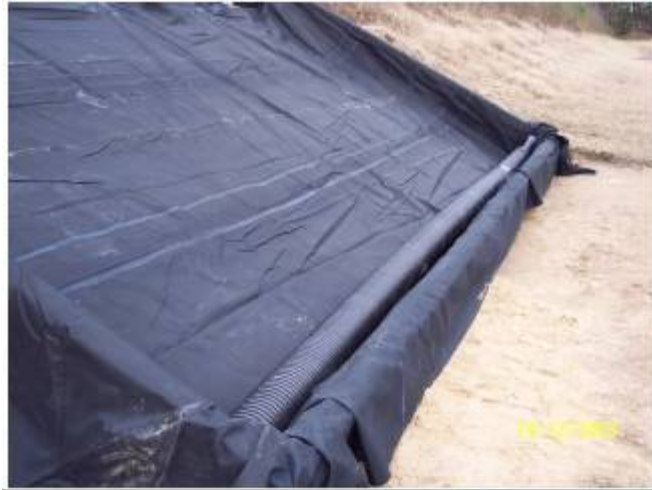
Figure 18. Water Collection Reservoir Installed.
