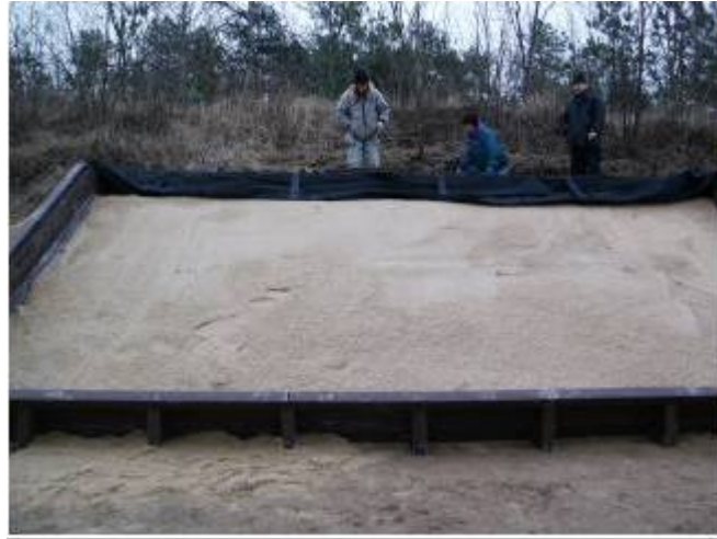
Figure 16. Laying the Bottom Rubber Liner.
