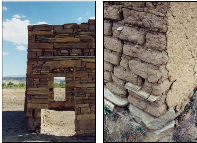
Figure 2.16. Pueblo Construction Materials. Pueblos were constructed of stone or adobe block depending on material availability (Ballweg, 2005).
