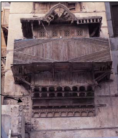
Figure 2.18. Plaster Erosion Control. Teak wood was placed between coral block and plastered over for erosion protection (King, 1998).
