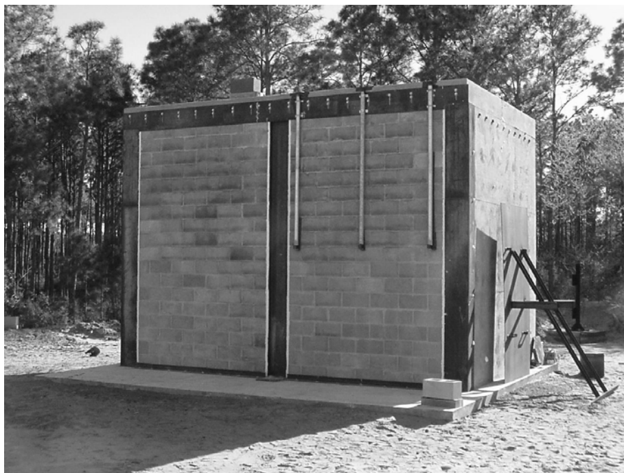
FIG. 4. Test Wall Setup
