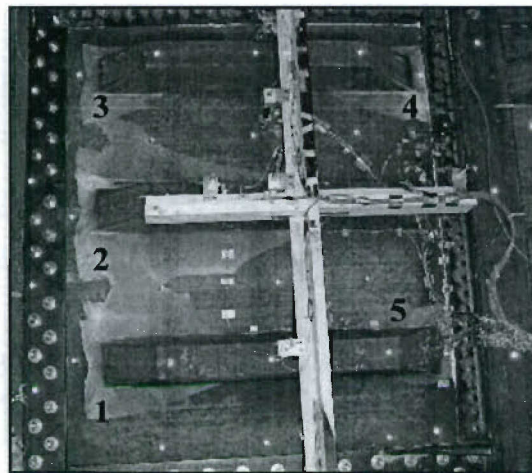
Figure 4.49. Stiffener Failure on P03
