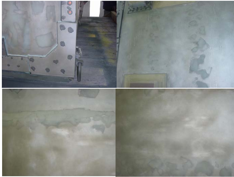
Figure 9. After wash primer.
