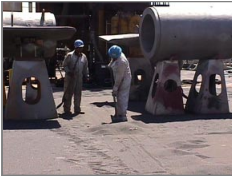
MANUAL CLEAN UP IS OFTEN PERFORMED ON GROUND
