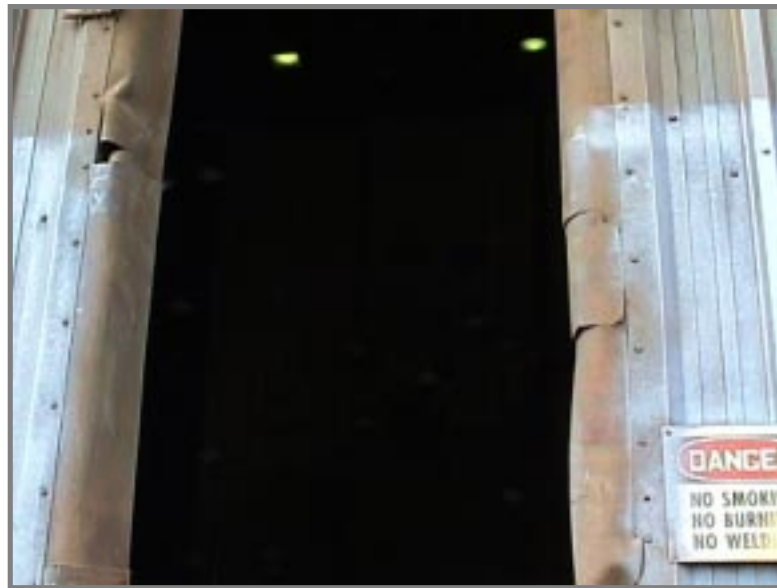
SHIPYARD BLAST AND PAINT HOUSE DOORS
