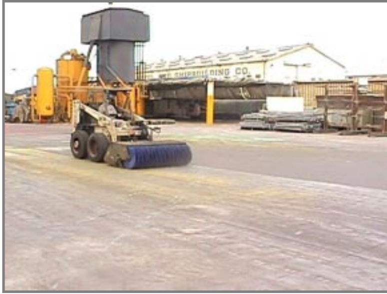
BOBCAT WITH POWER SWEEPER ATTACHMENT COMPLETING SPENT GRIT CLEAN UP
