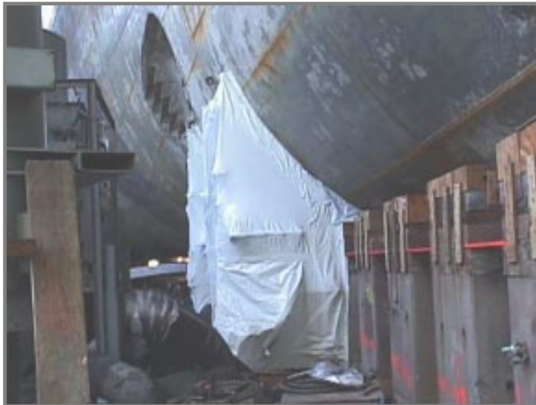
TYPICAL LOCALIZED CONTAINMENT (SHRINK WRAP) IN DRY DOCK
