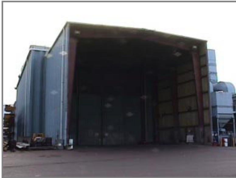
THE SHIPYARD BLAST HOUSE
