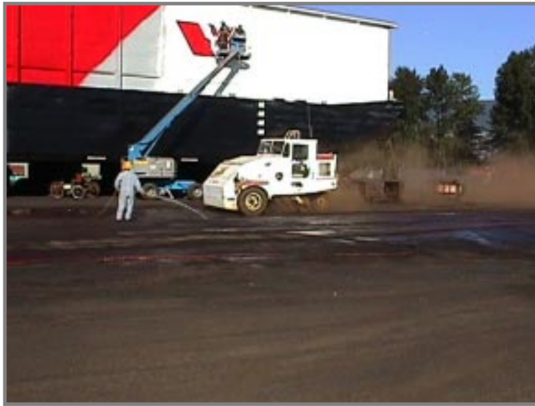
UNSEGREGATED PAINT AND GRIT CLEAN UP OPERATIONS
