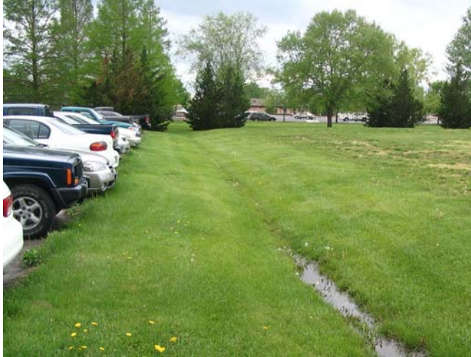
View facing west from the southeast corner of the site of the Proposed Action. The drainage swale is visible in the foreground.
