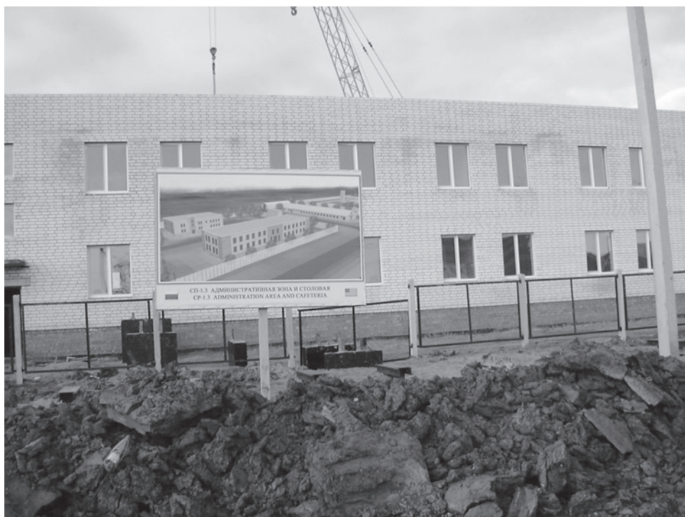
Figure 3: Administration/Cafeteria Building under Construction, November 2005
