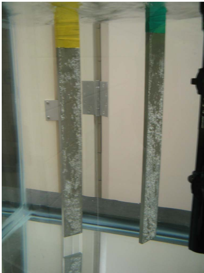
Figure 183. Yellow notchless and green notched beam in the tank. Visible salt deposits in under 24 hours.
