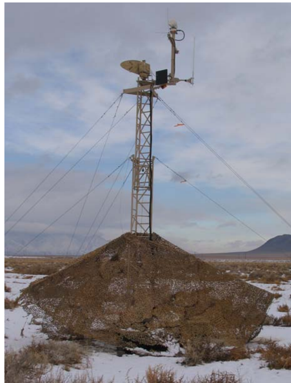
Figure 12: Remote Sensor Station (RSS).
