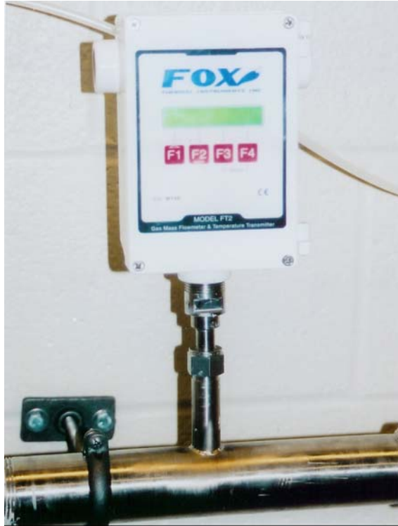
Figure 6 Fox Thermal Instruments FT2 Flow Meter
