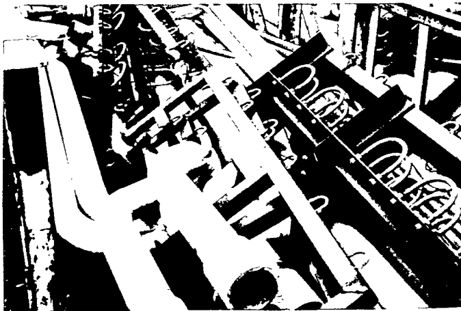
FIGURE 5-34: Subcontractor provided pipe supports which have galvanized U-bolts temporarily attached for ease of in-process material control.
