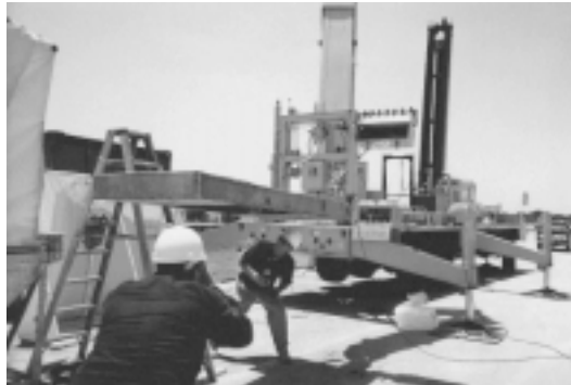
Figure 4: Temporary Extension Bracket Used for Demonstration Exercise
