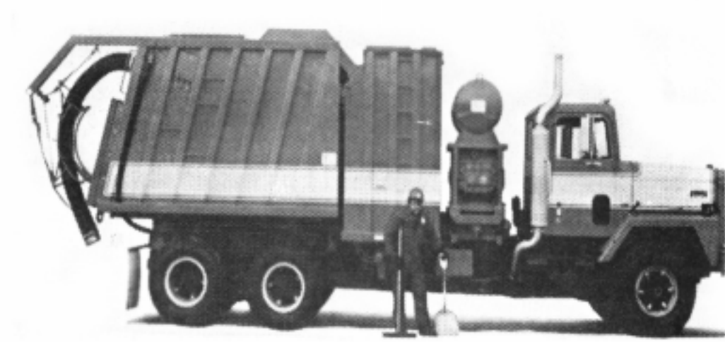
Figure 3-6: Mobile Vacuum Recovery Truck with Single-Chamber Collection Tank
