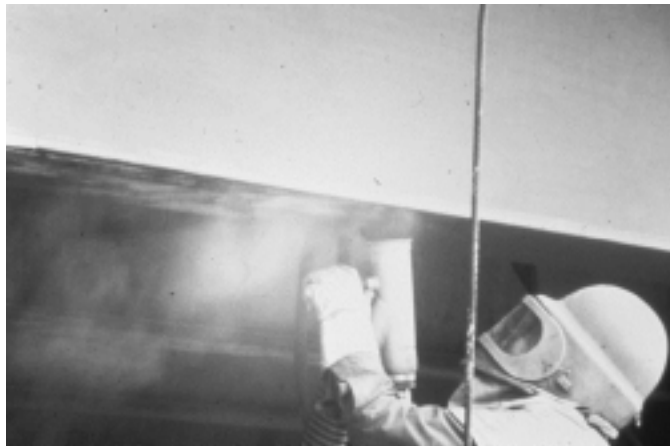
Figure 4-2: Vacuum Blasting Demonstrating Poor Seal (SSPC File Photo)
