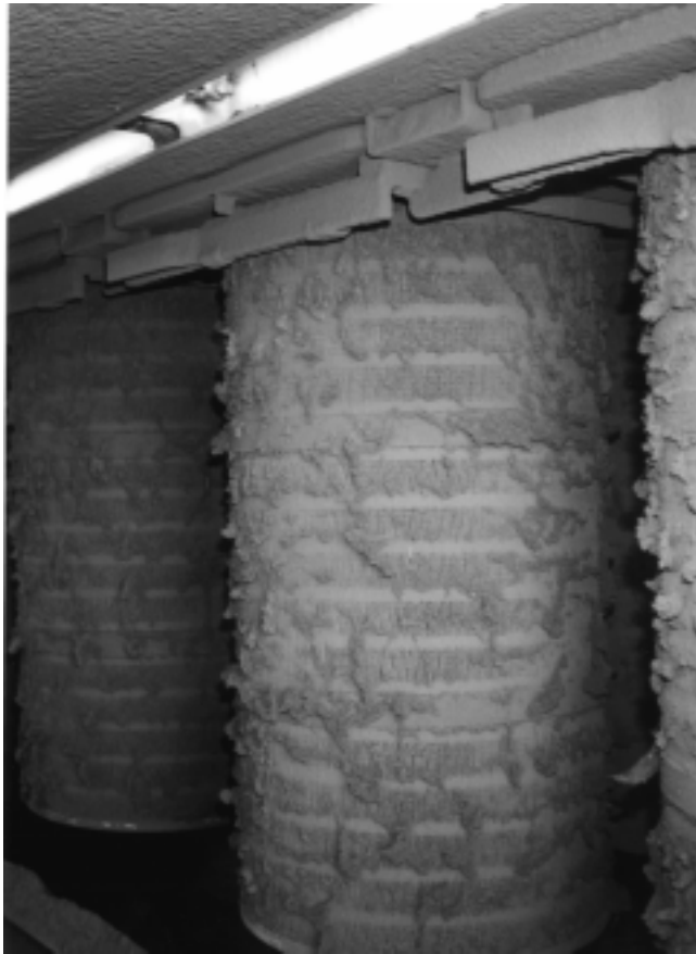
Figure 7-1: Dry Cartridge Filter Ready to be Replaced (Courtesy of Todd Shipyard)
