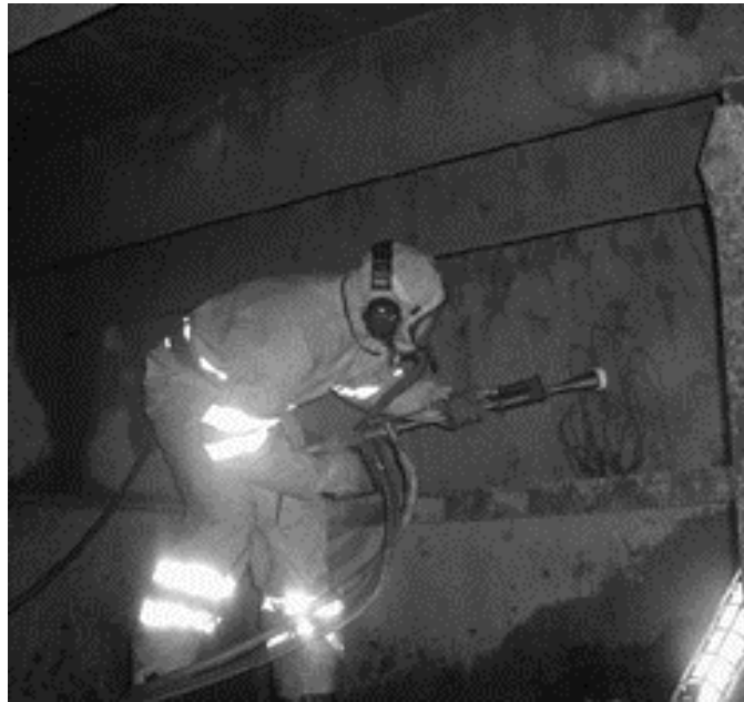
Figure 4-8: Water-jetting aboard ship (Courtesy of Hempel Coatings)
