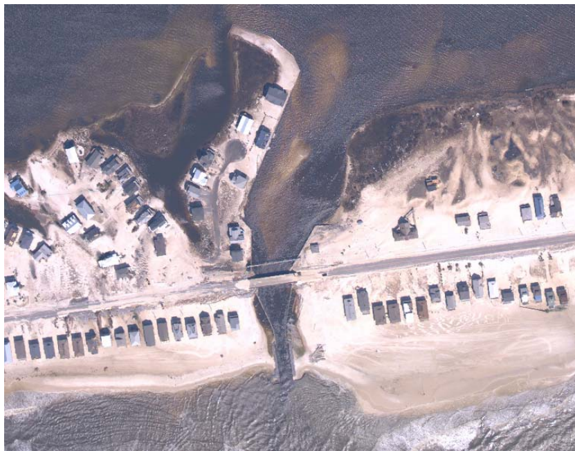
Figure 38 (2004 post-Hurricane Ivan aerial photos of Little Lagoon Pass)
