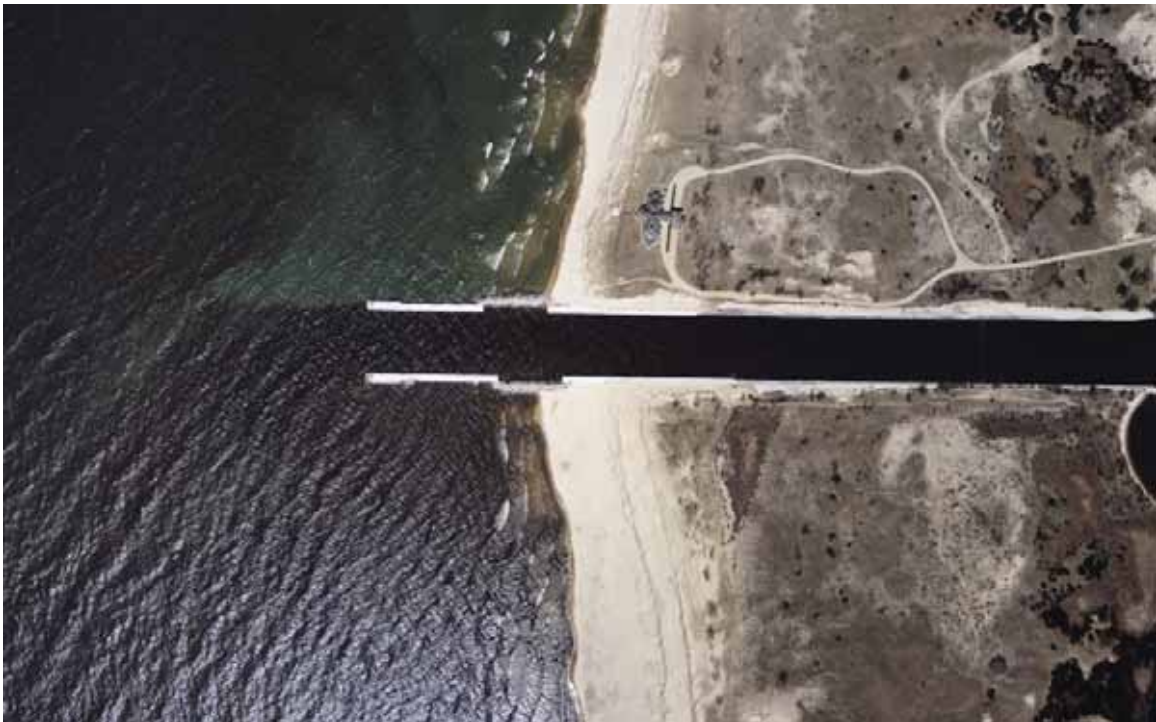
Figure C1. Aerial view, Saugatuck Harbor, MI.
