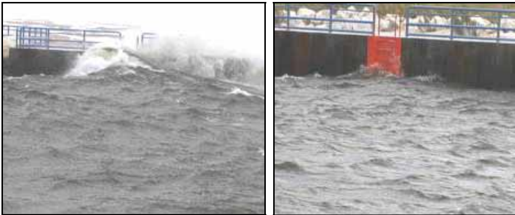
Figure 3. Waves along south jetty and entrance channel, Pentwater, MI, June 1999, looking south from north jetty: a) waves lakeward of pocket; b) waves attenuated landward of pocket (from Dr. Donald D. Carpenter).
