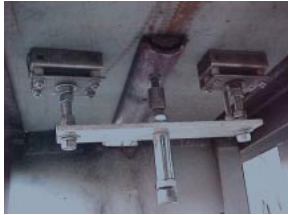
FIGURE 3-5 CLAMP ASSEMBLY SUPPORTS TROUGH
