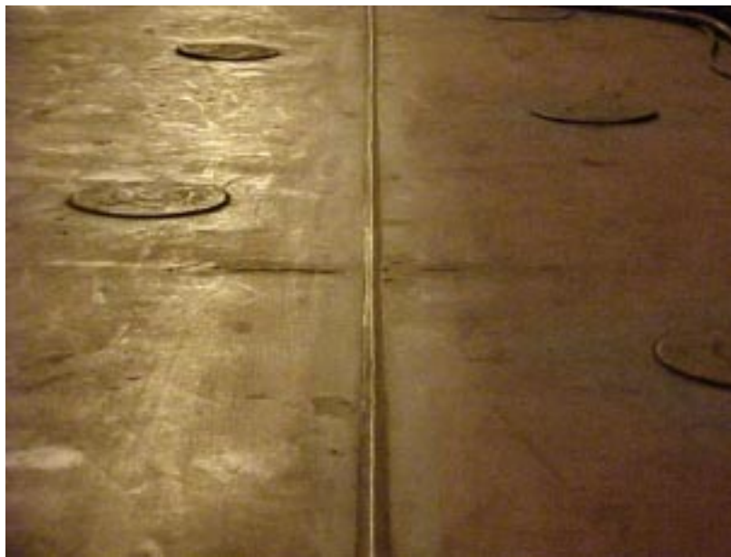
MRF Face Reinforcement -- Blocks 241 / 243
