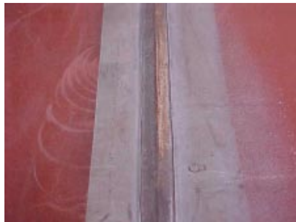
MRF Face Reinforcement -- Blocks 313 / 395
