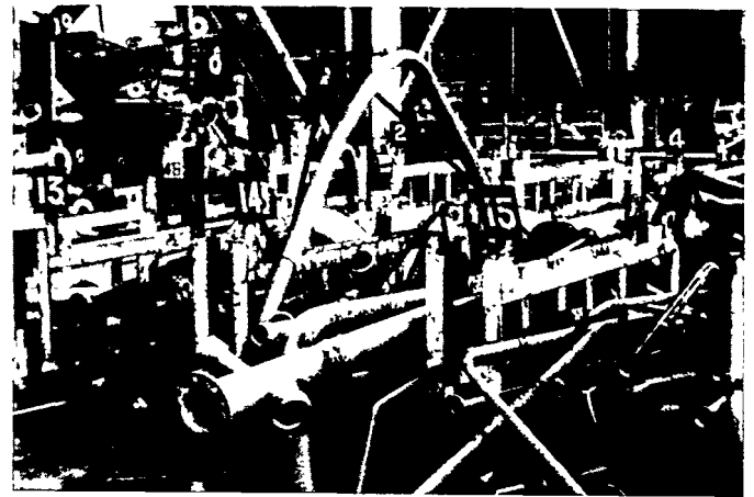
FIGURE 5-12: Outfit palletizing utilizes standard containers which may easily be handled by crane or forklift. In shipyards where zone outfitting is practiced, significant yard areas are devoted to sorting and storing (often on multi-tiered levels) palletized material.
