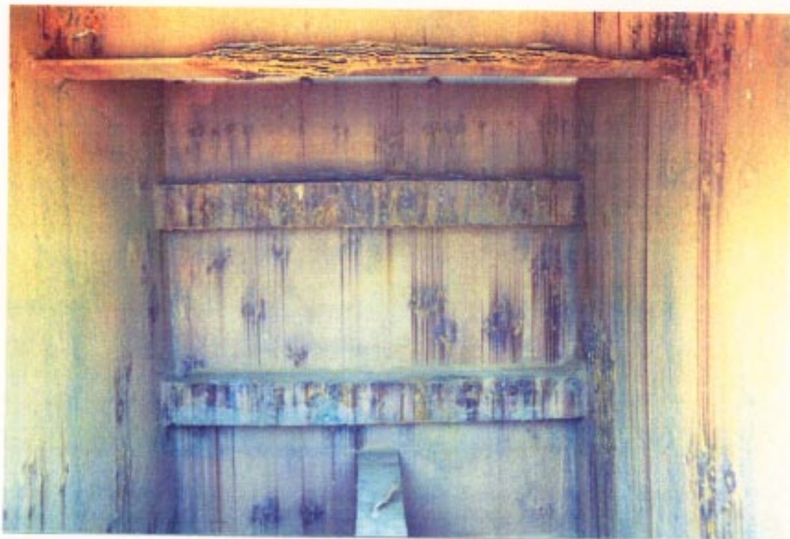
PHOTOGRAPH 6-SURFACE TOLERANT EPOXY A OVER HAND TOOL CLEANED SURFACE
