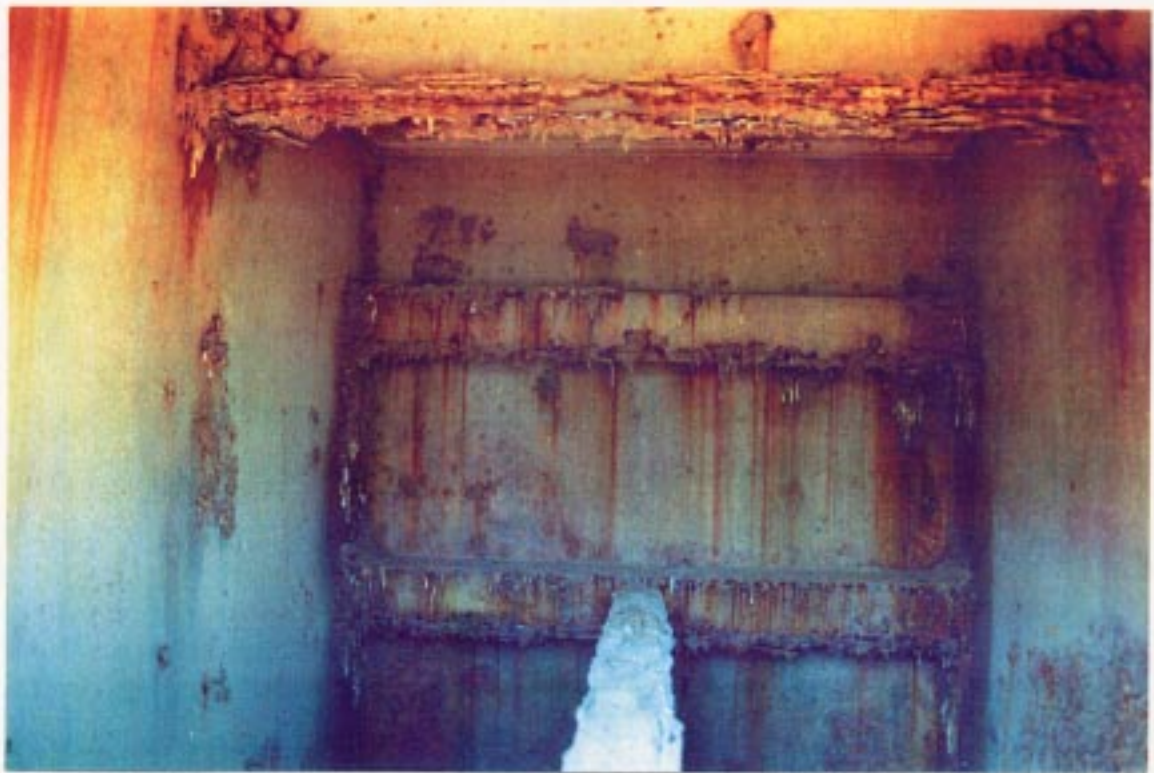
PHOTOGRAPH 10-AGED EPOXY WITH ADDED ZINC ANODE
