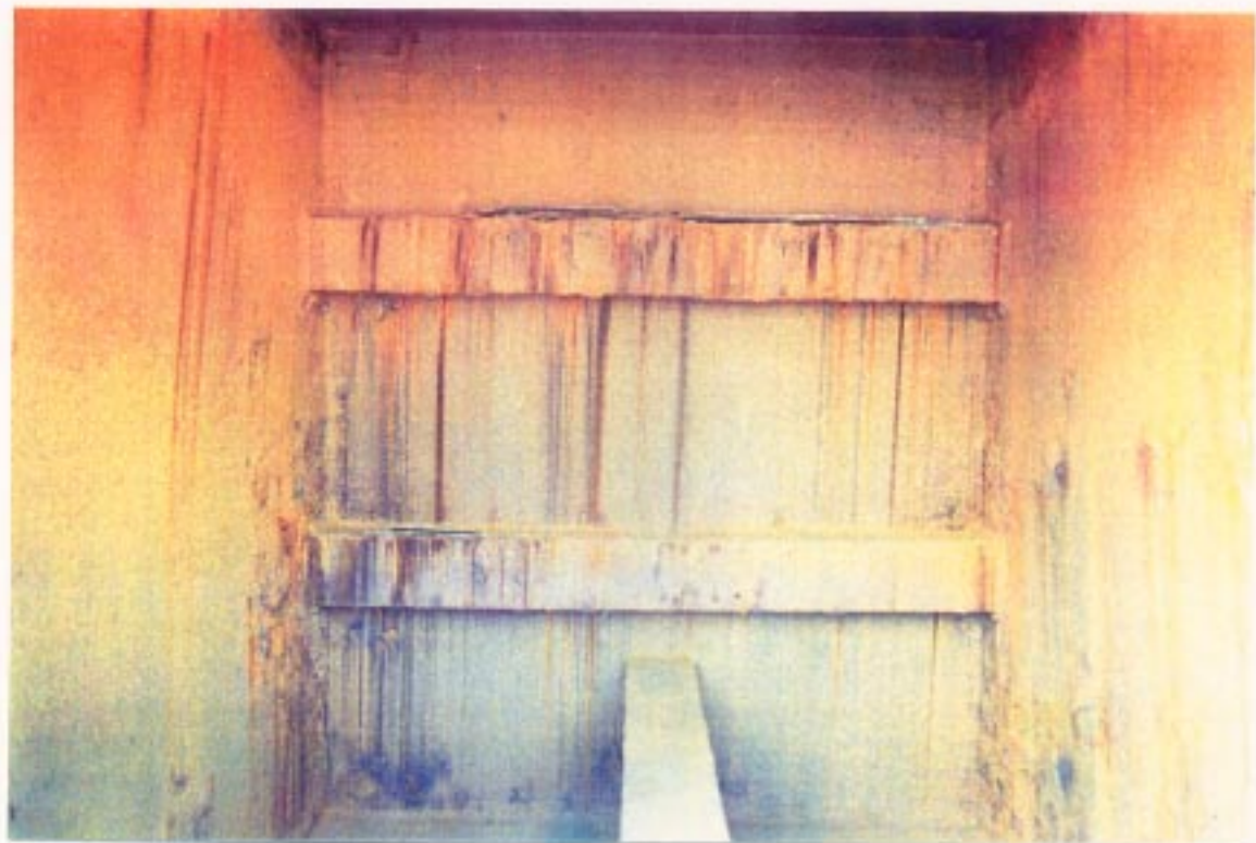
PHOTGRAPH 8- SURFACE TOLERANT EPOXY B
