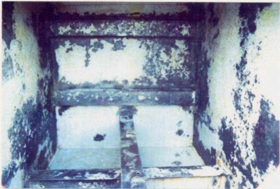
PHOTOGRAPH 2A- SWEEP BLAST CLEANED SURFACE
