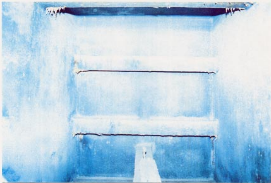
PHOTOGRAPH 12- SOLVENT BASED INORGANIC ZINC WITH ZINC ANODE
