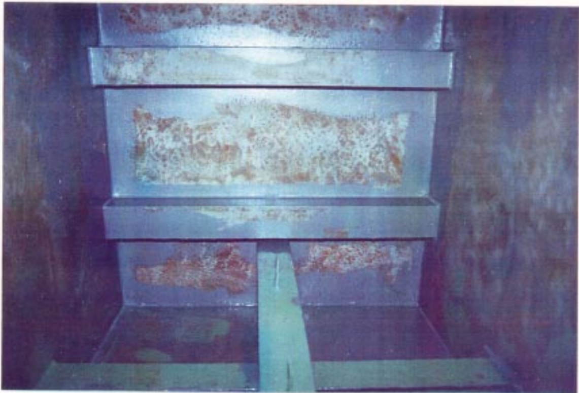
PHOTGRAPH 5- STRIPE COATING BETWEEN COATS
