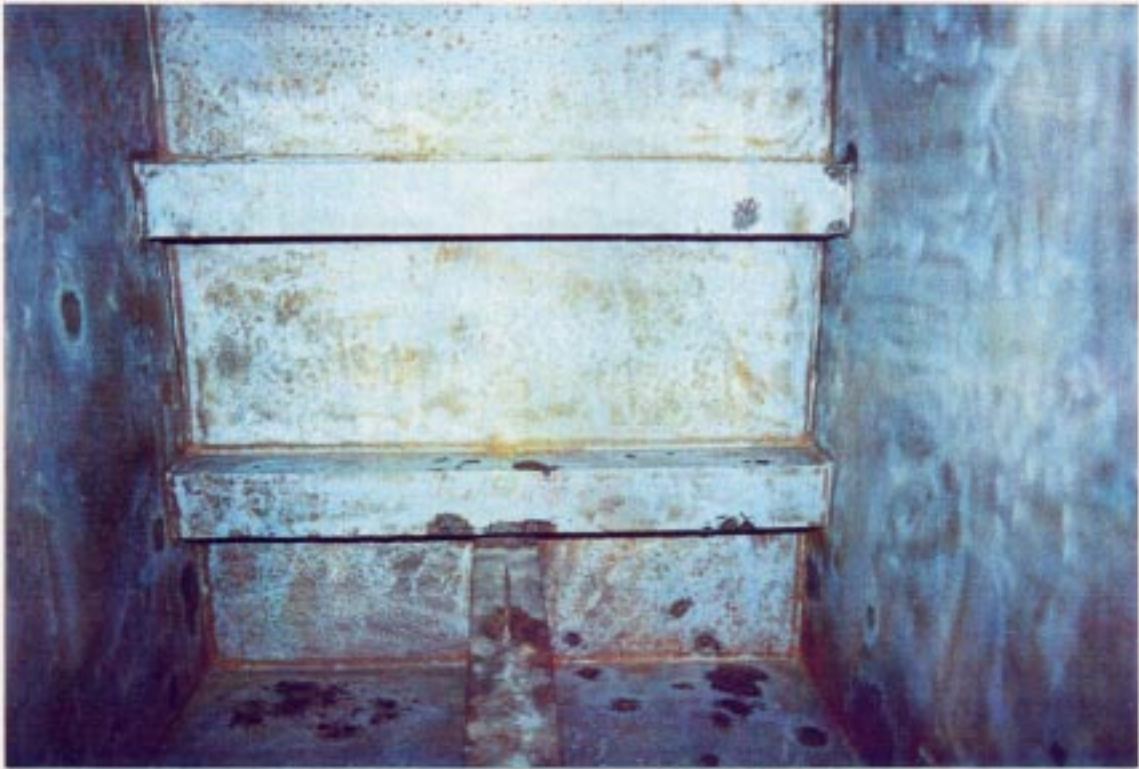
PHOTOGRAPH 3- REPAIR SURFACE PREPARATION TO MIL-P-24441
