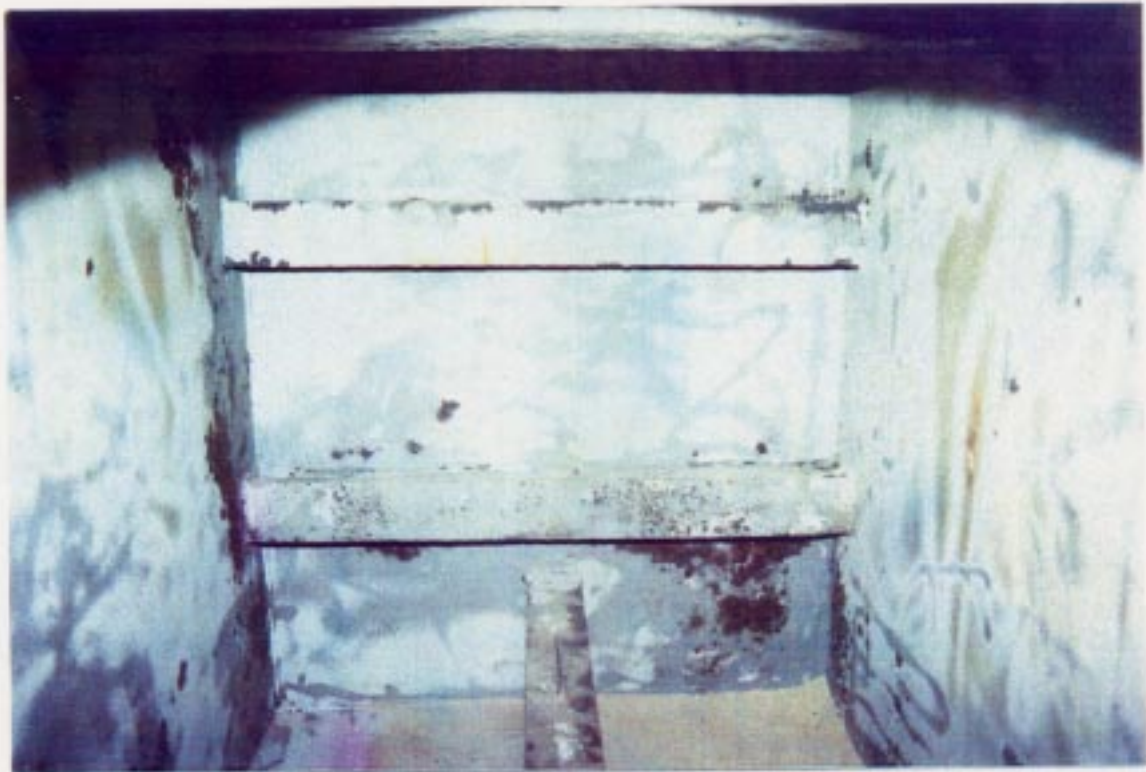
PHOTOGRAPH 2A- SWEEP BLAST CLEANED SURFACE
