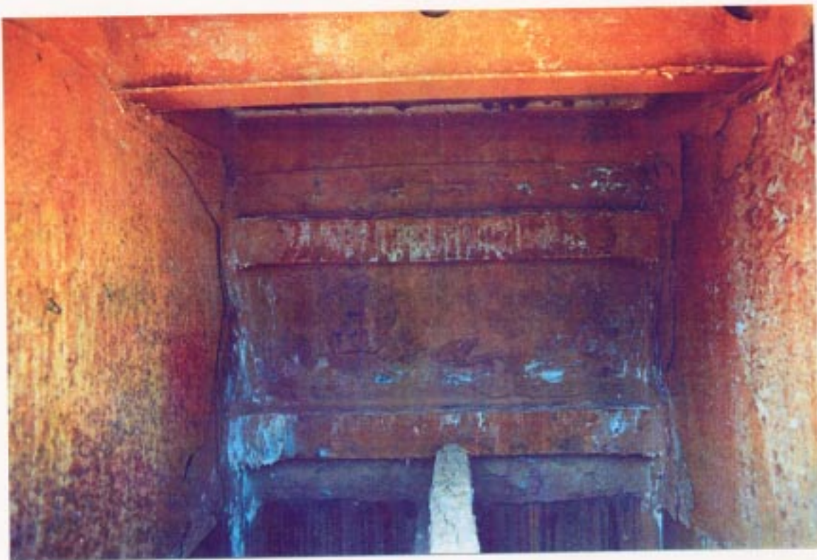
PHOTOGRAPH 11- PARTIAL COATING WITH ZINC ANODE
