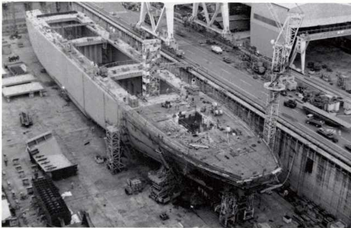
FIGURE 3-50: Erection Level. Keel laying plus 24 workdays.
