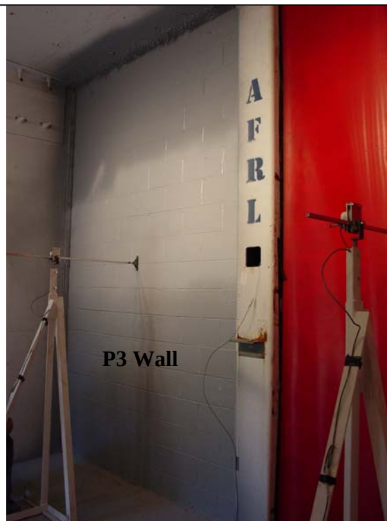
Figure 5.26 – CMU Wall with P3 Polymer Retrofit
