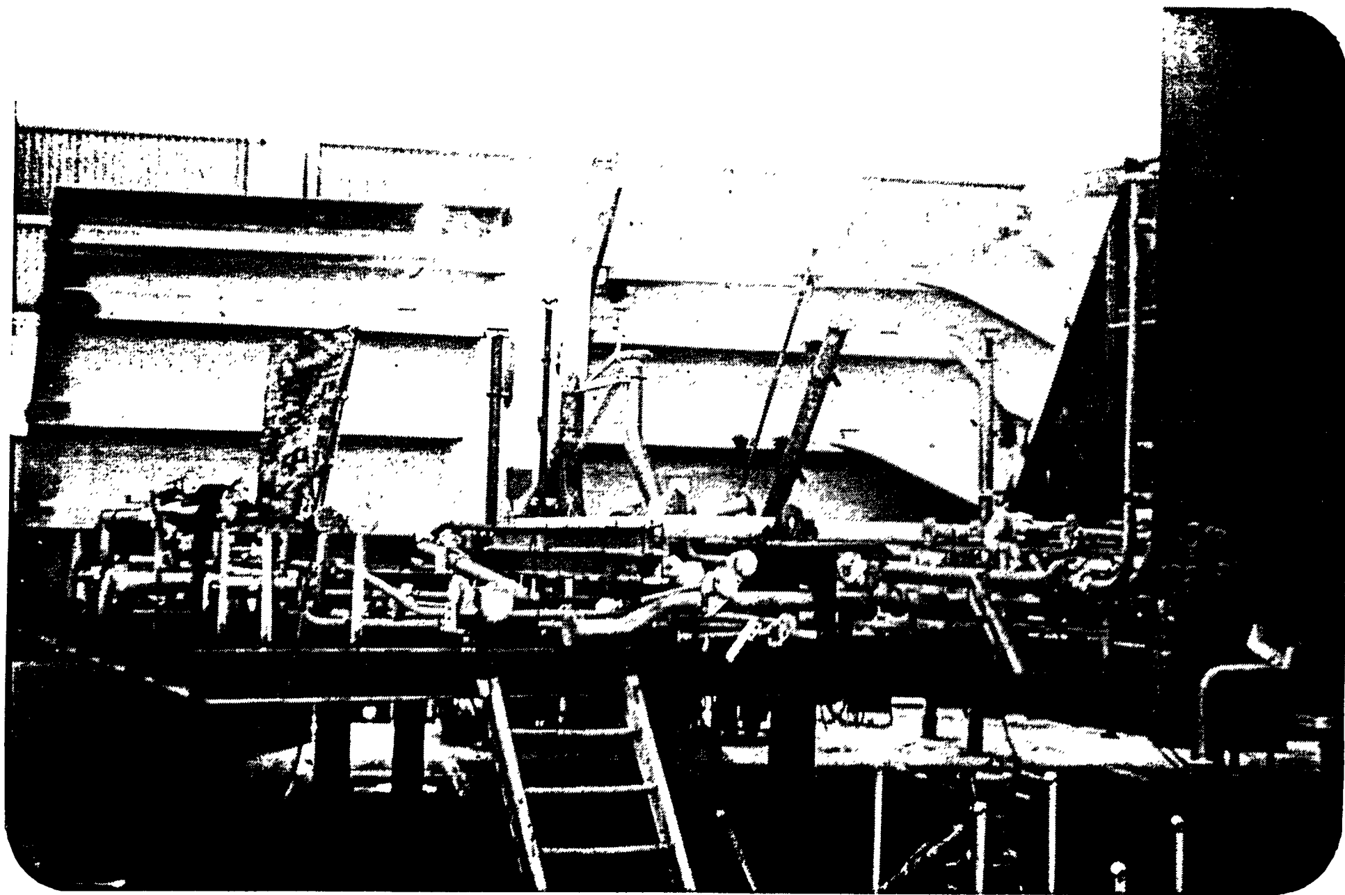
Curved panel structural block outfitted upside down. IHI. Aioi..
