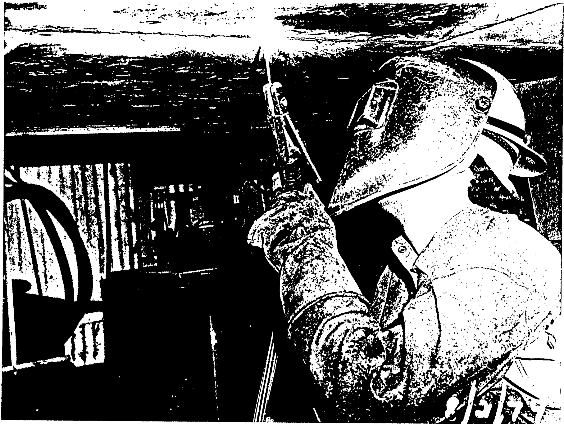
Fig. 27 shielded metal-arc welding in the overhead position.
