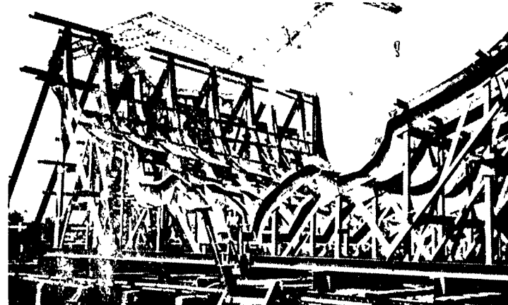
4.n Fixed Jig used for Block Assembly of Navy Ship
