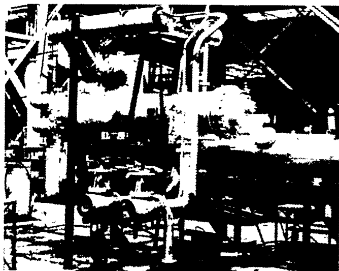
FIGURE 1-4: A functional unit consists mainly of components necessary for the operation of something, e.g., a heat-exchanger assembly. It is generally associated with one system.
