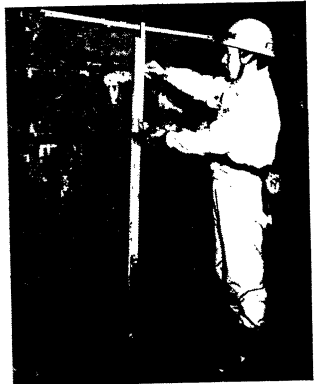
FIGURE 6-15: Specific A/C procedure apply to: A. Checking a measurement between panel and bracket edges in a sub-block. B. Checking a measurement between the edges of a panel and internal structure in a block. C. Checking alignment of a tank-top panel relative to a bottom-shell panel in a block. D. Monitoring bottom alignment between keel laying and launching. The distance measured is that from the bottom shell to a reference line marked on the vertical angle-iron which is fixed to the dock floor.
