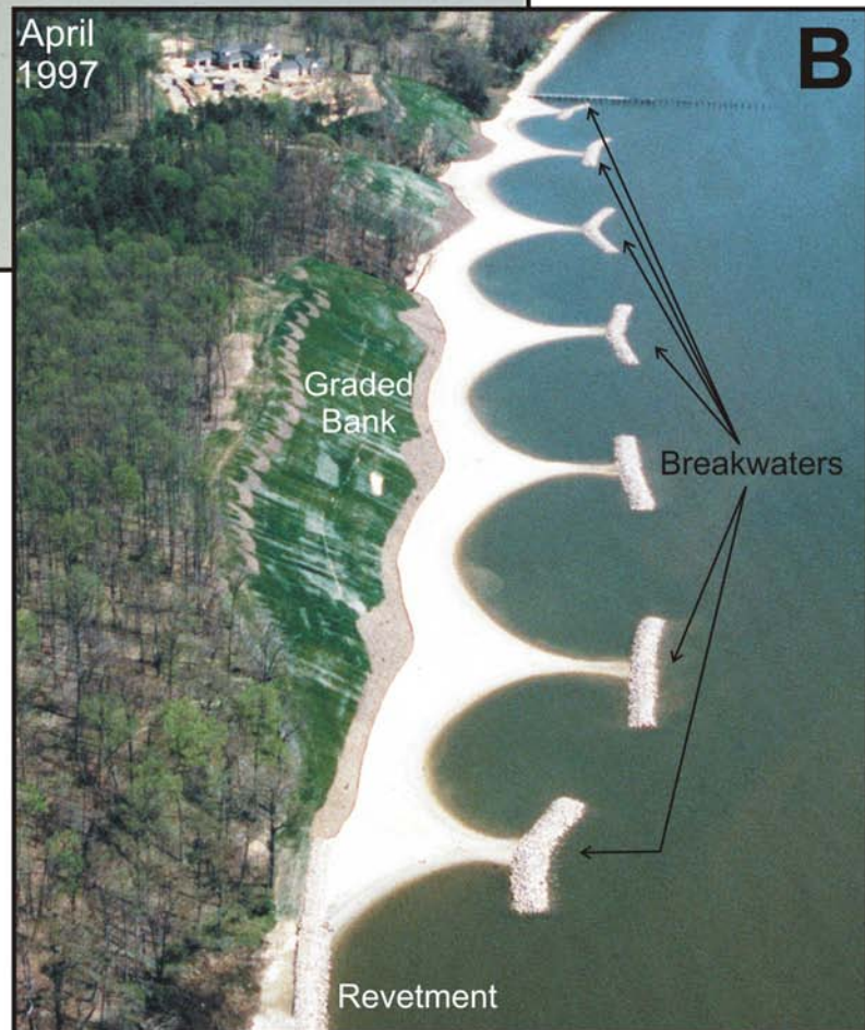
b. After installation
