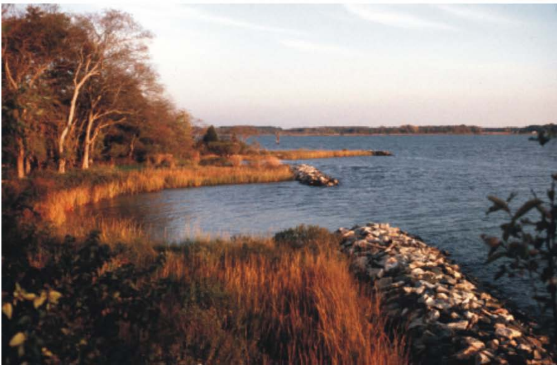
Figure 5. Stone sill connecting breakwaters with sand fill and marsh implantation on Choptank River, Talbot County, MD, just after construction and 5 years post-construction (Hardaway and Byrne 1999)
