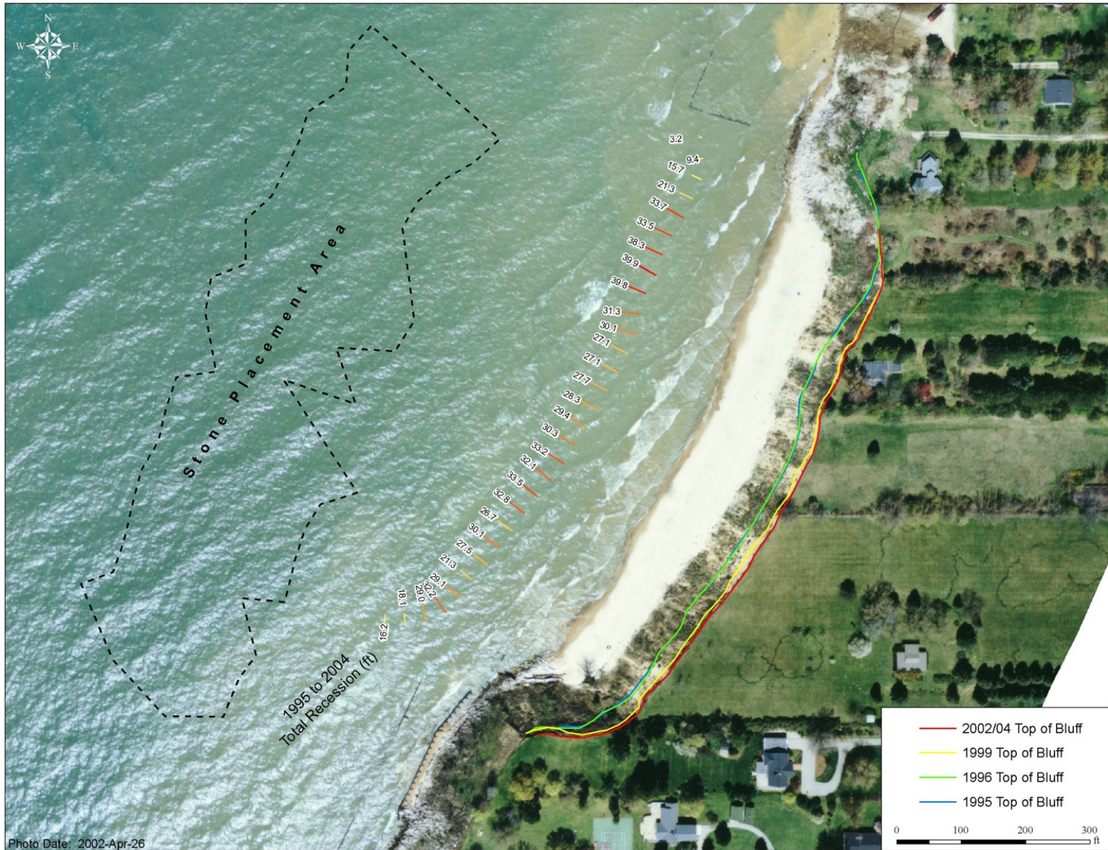
Figure 5. Bluff recession at Shoreham, MI, between 1995 and 2004.
