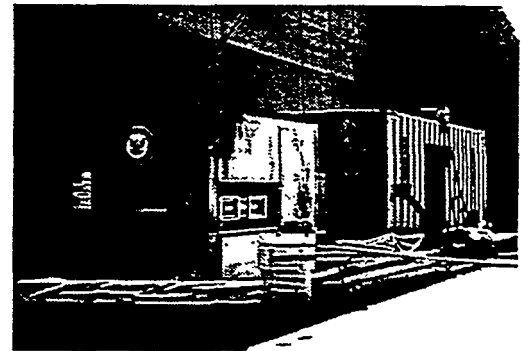
Figure 9 Pump and Recovery Subsystem Trailer
