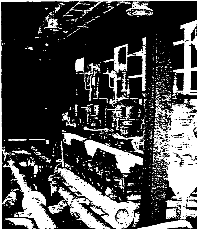
Figure 8 Outfit Unit Installed On-block before Erection
