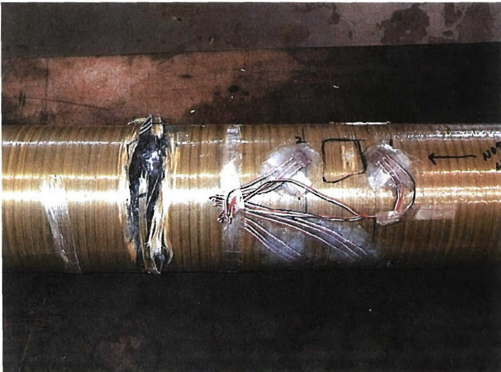
FIGURE D-15. Failure Photograph 2.
