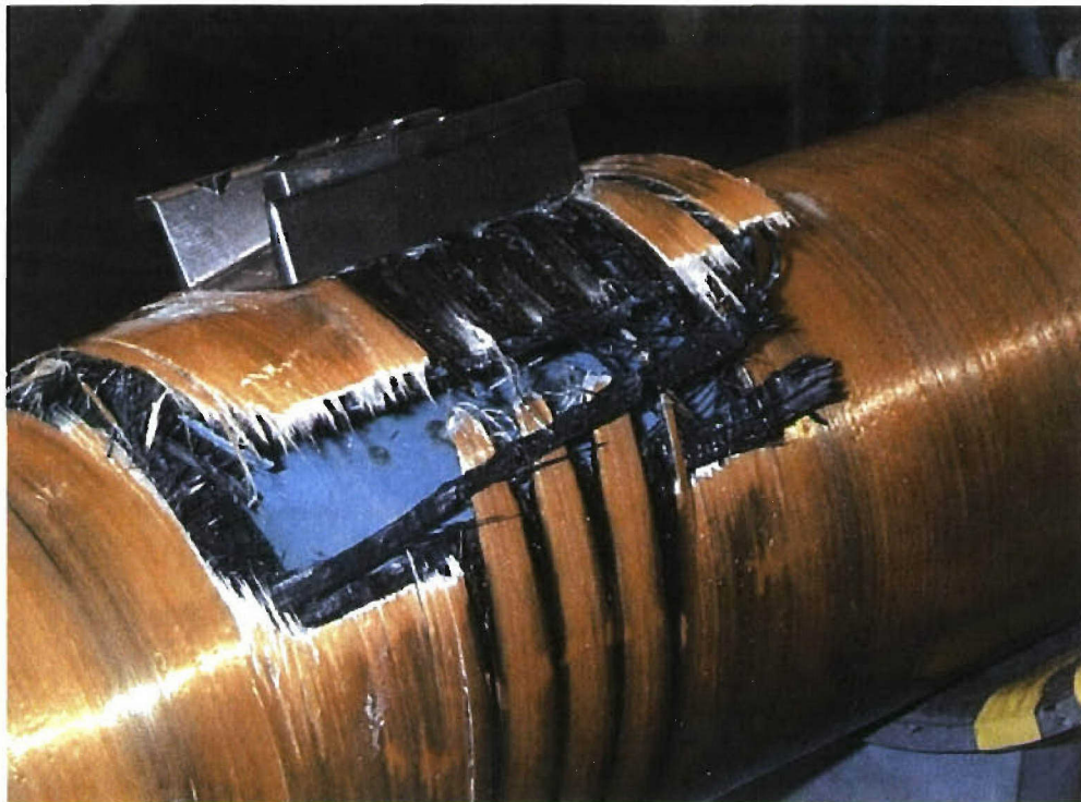
FIGURE H-12. Middle Hanger Failure (With Release), Outside View.
