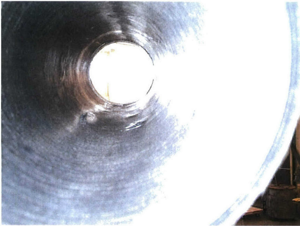
FIGURE J-9. Middle Hanger Failure (No Release), Inside View.
