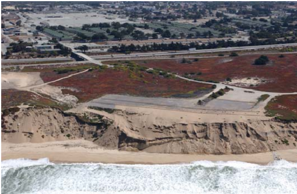
Figure 3. Photo of the Stillwell Hall site taken October 11, 2004 showing erosion of the peninsula on which the now demolished structure used to stand.
