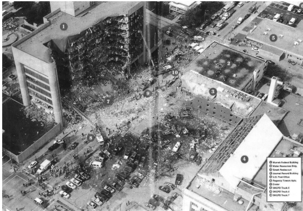
Figure 8. Alfred P. Murrah Federal Building, 19 April 1995
