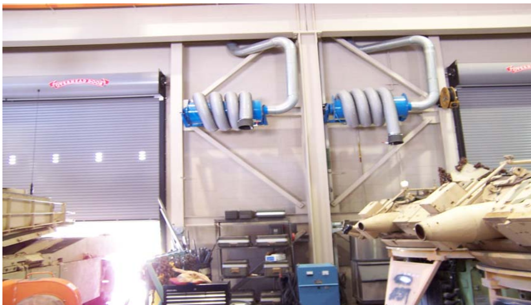
Figure 38. New individual vehicle exhaust with spring recoil hose reels.
