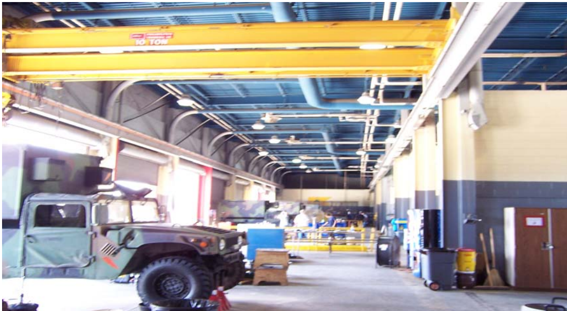
Figure 37. Maintenance Shop with old central vehicle exhaust.
