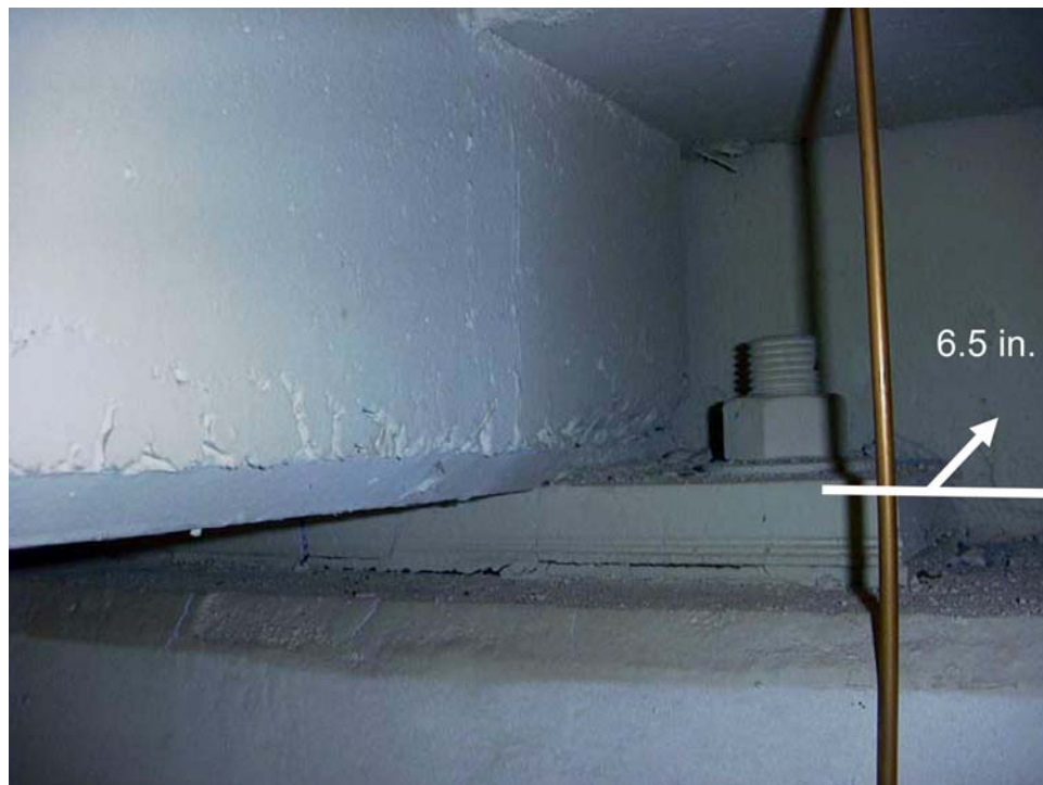
Figure 1-10. Downstream T-beam connection: T-beam bearing plate rests on Neoprene pad, bolt through plate with slotted holes (an ideal roller condition). Note: The slot is assumed to permit less than 1 in. of free travel in each direction. The free travel length is estimated on the assumption that the washer shown in the figure completely conceals the slot.
