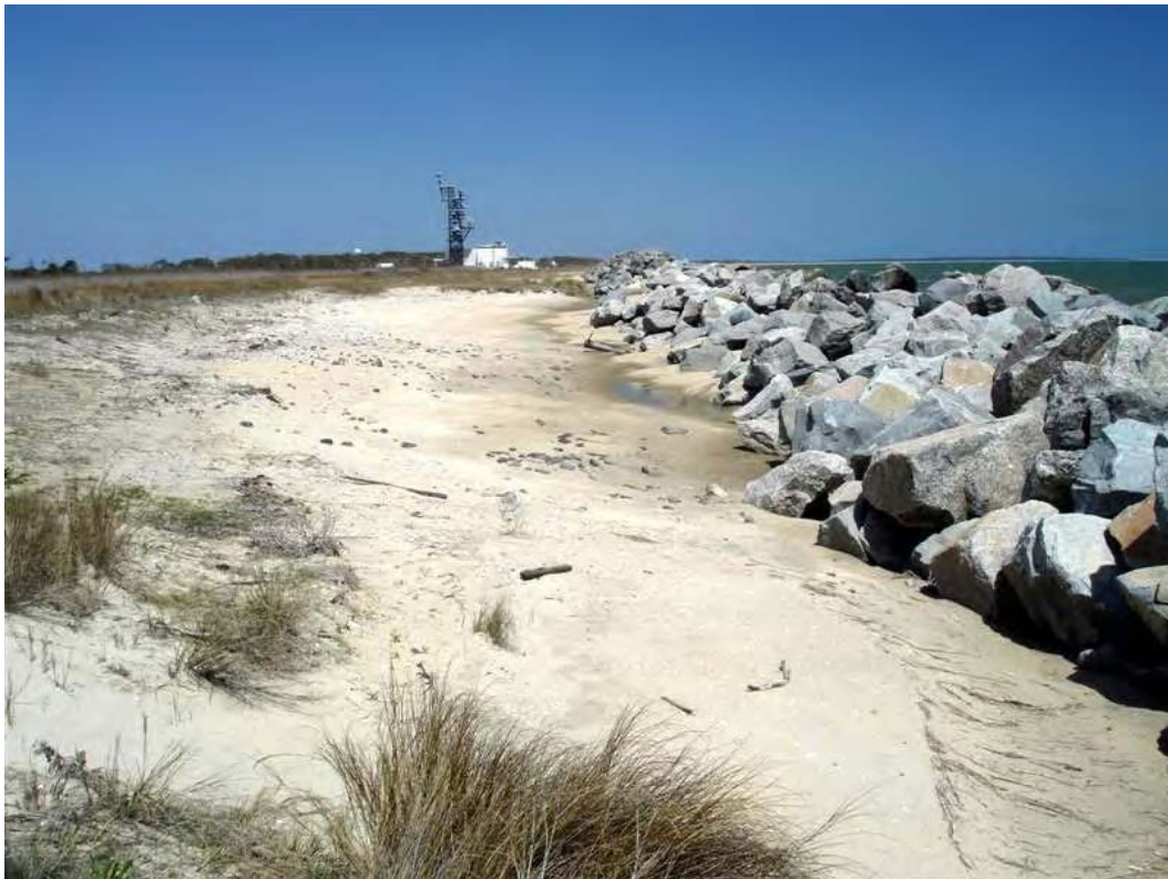
Figure 21. View north from U.S. Navy Aegis facility (Building V10/V20) toward Building V-24, 18 April 2006. Sand has been lost through seawall, and lowest areas contain standing water even on a calm day.
