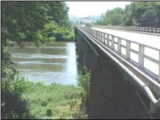
Downstream Side View (7/23/03)
