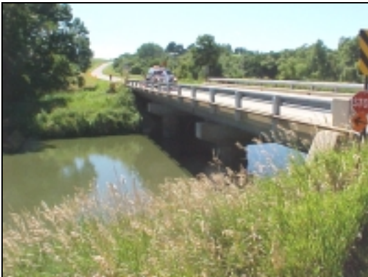
Downstream Side View (7/15/03)
