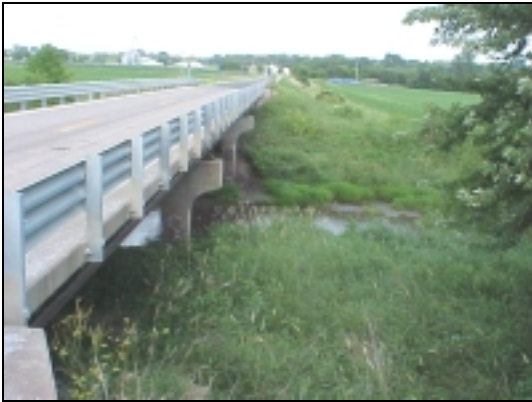
Downstream Side View (7/17/03)
