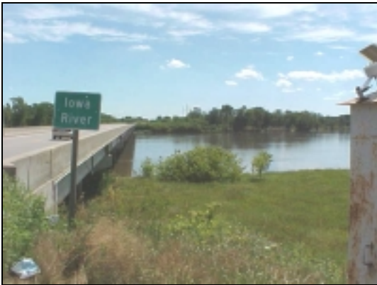
Downstream Side View (7/24/03)
