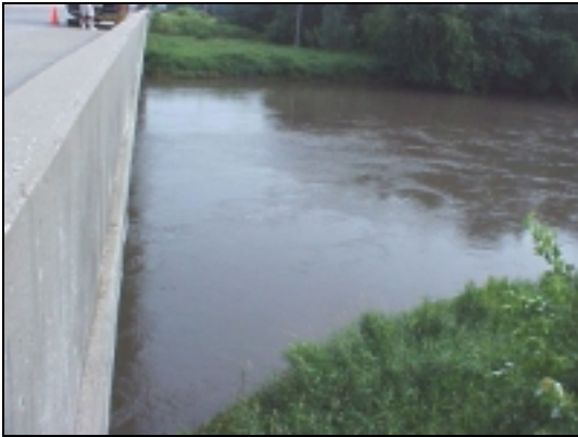
Downstream Side View (7/18/03)
