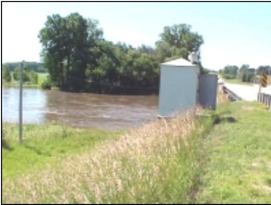
Downstream Side View (7/11/03)
