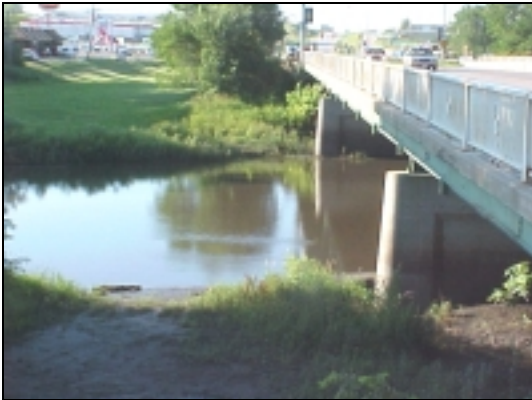
Downstream Side View (7/16/03)
