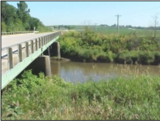
Downstream Side View (7/23/03)
