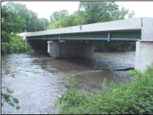
Upstream Side View (7/17/03)
