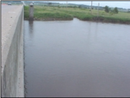
Upstream Side View (7/18/03)
