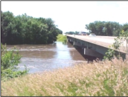
Downstream Side View (7/11/03)
