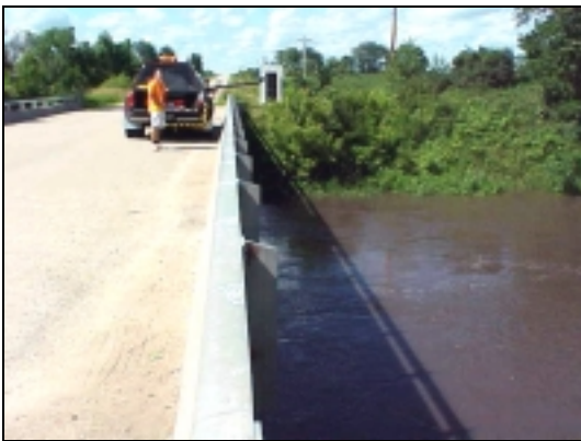
Downstream Side View (7/10/03)
