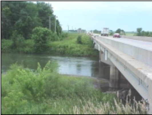
Downstream Side View (7/16/03)
