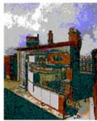
Viewing gallery with advanced glazing in all windows. On/off lighting control, EE lighting. TIM wall. PV hybrid + ducted wind turbines
