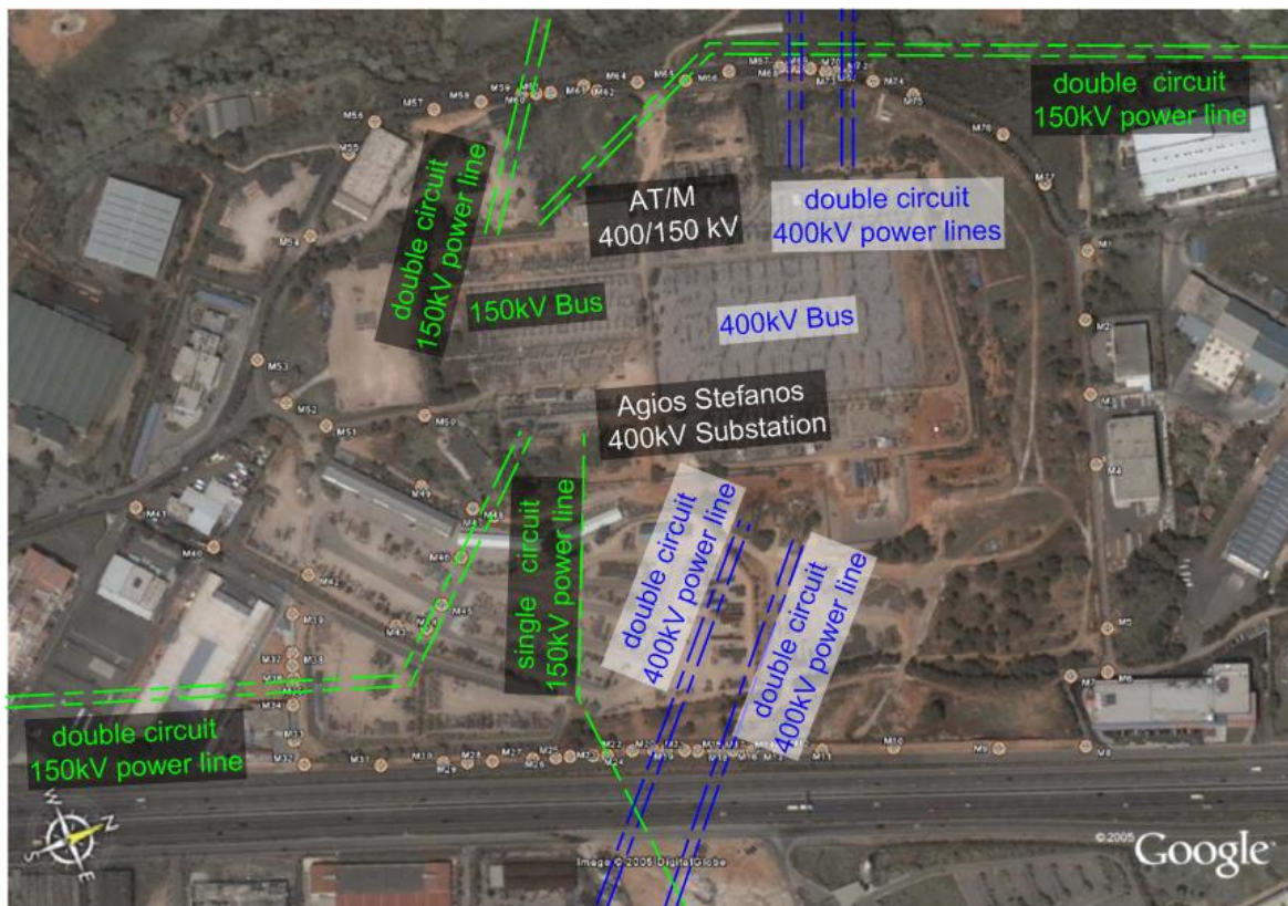
Fig. 6. Satellite photo of Agios Stefanos 400kV substation (Greece) where the routes of 150kV and the 400kV power lines connected to it and the locations where EEAE have conducted measurements outside its perimeter are indicated.
