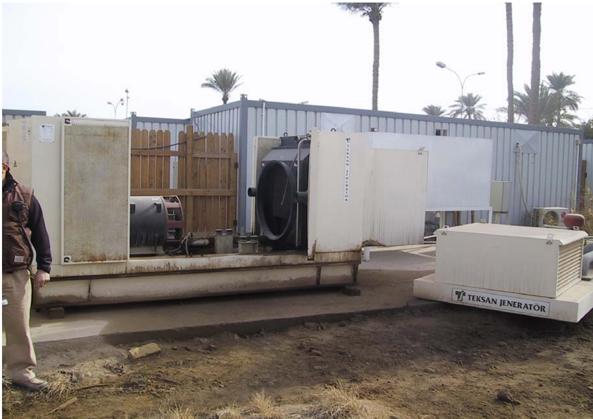
Photo 1. Shell for the 500-Kilowatt Generator Undergoing Repairs
